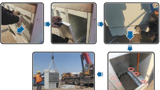
Figure 6-74 Removing the old ring main unit
