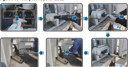
Figure 6-68 Pulling out AC power cables
