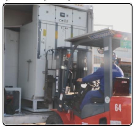
Figure 6-73 Removing the old ring main unit
